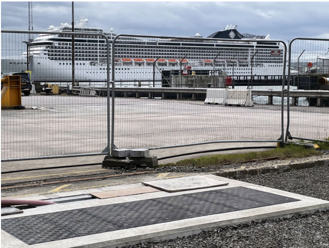
Custom Fibrelite trench access covers with hot dip galvanised steel frames
