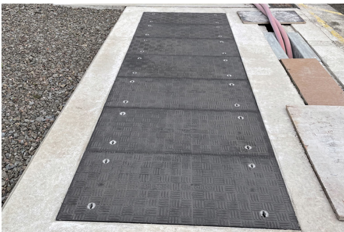
Trench covers were stepped 117 to 150mm deep to achieve the required F900 load rating
