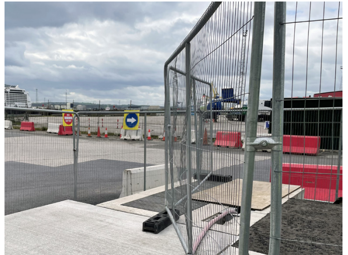
F900 (90-tonne) load rated covers were required
