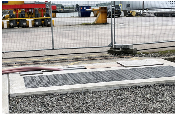
Fibrelite covers are lightweight, suitable for easy/safe manual removal
