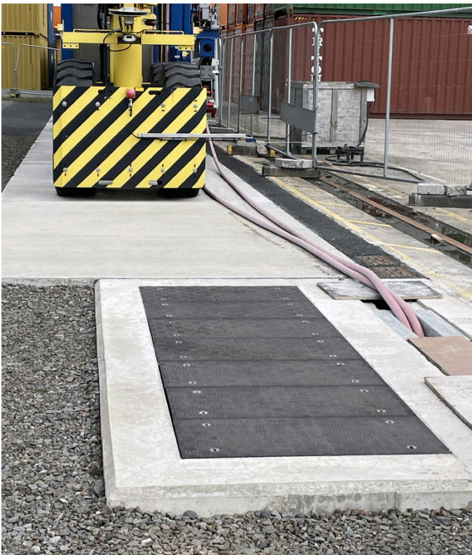
Lightweight Fibrelite F900 trench covers over cable anchor pits
