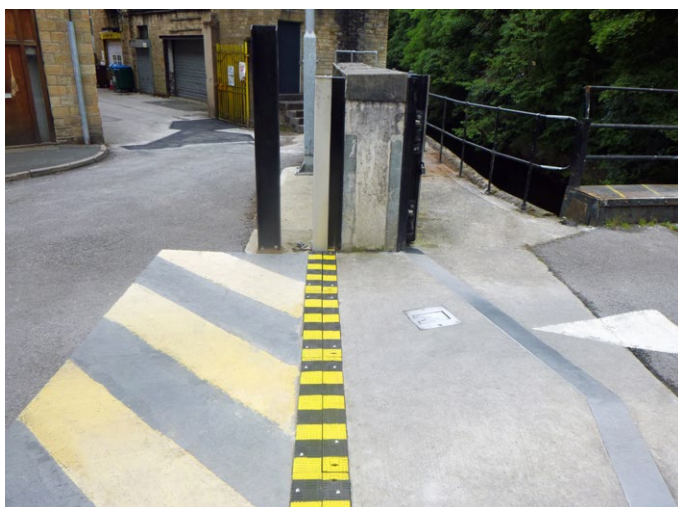
Fibrelite retrofit replacement GRP composite trench access covering solution
