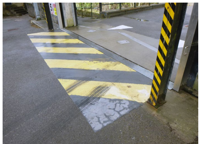
The site approached Fibrelite for a long-term retrofit replacement
