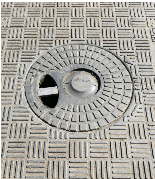
FL90CD With Embedded RF Antenna
