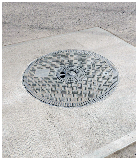
Radio Frequency Friendly Cover Installed by US Water Utility Company
