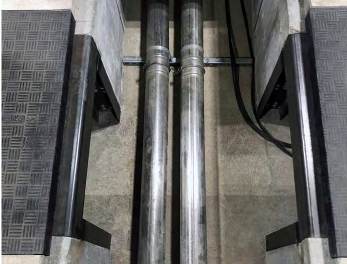
I-Beams allow for coverage where no seating faces are available
