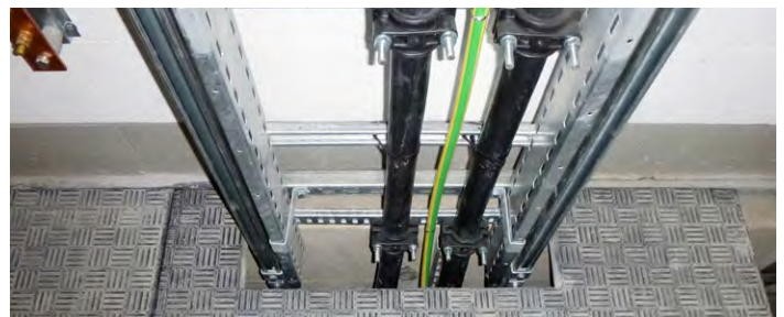
Field cut slots created on-site
