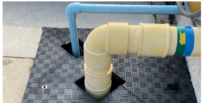
Factory cut cover openings
