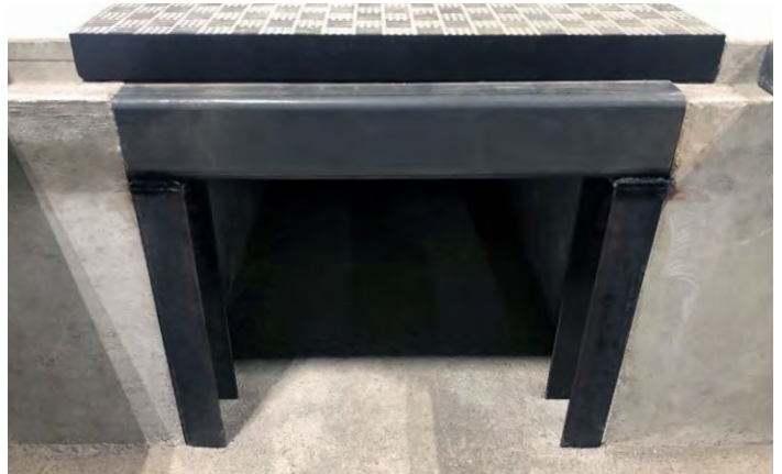
Example of I-Beam support at a junction
