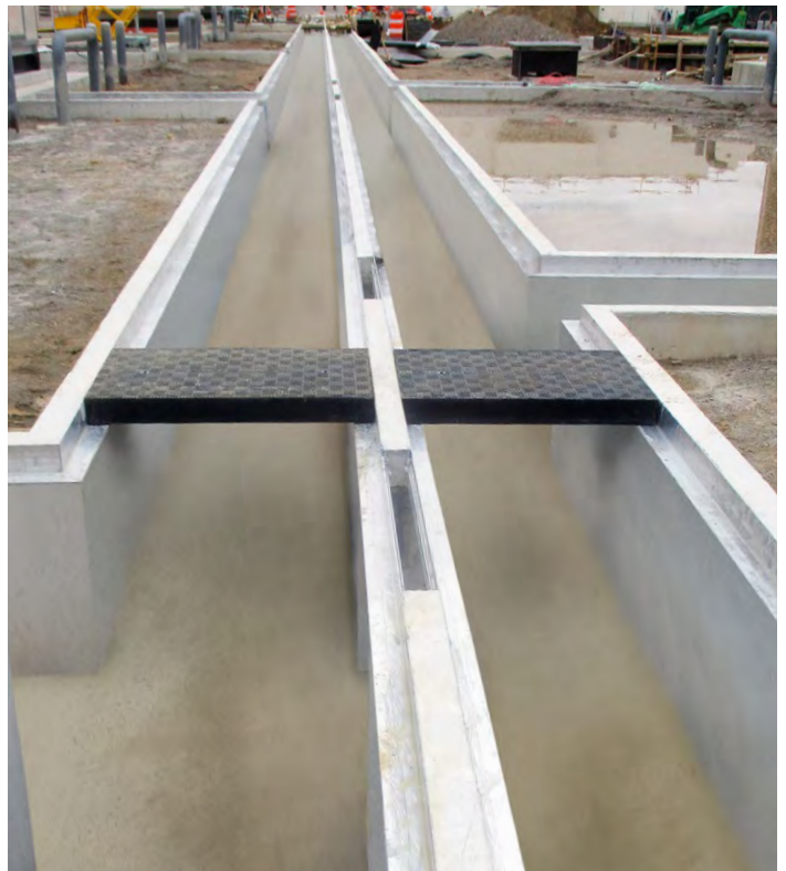
Center support providing the seating face for covers
