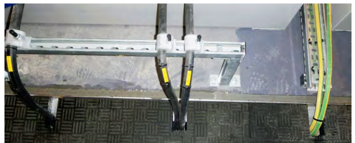
Field cut slots for pipe and cable penetrations
