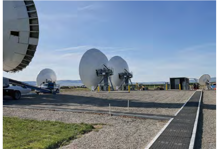
Fibrelite trench covers installed in Trenwa precast trench at a mission-critical satellite facility
