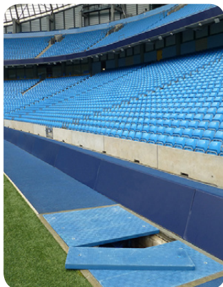
Heavy corroding steel covers requiring a crane & dedicated lifting equipment
