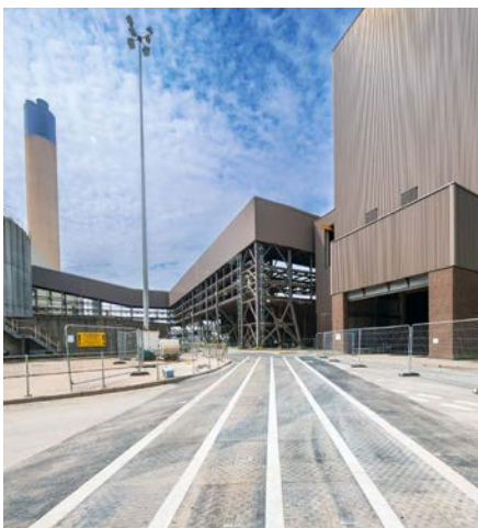
D400 load rated trench covers (in line with the BS EN 124 load classification)
