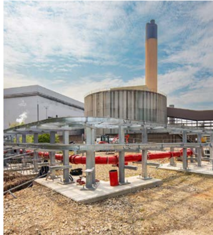
A GRP trench covering solution was for easy safe manual handling
