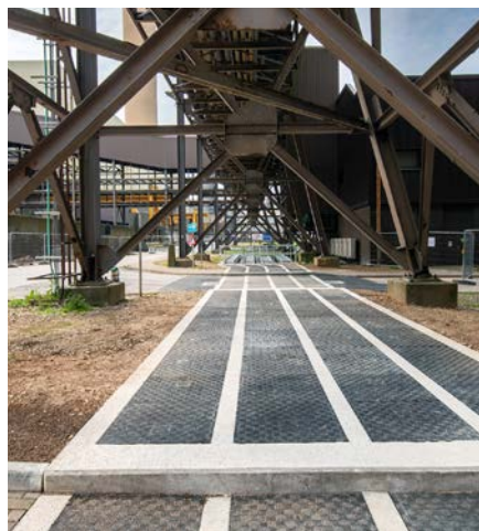
625 metres of custom GRP trench cover were designed & manufactured
