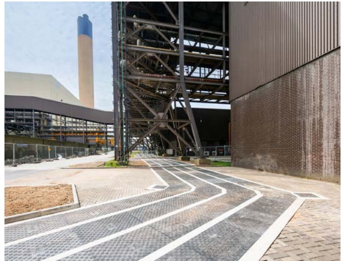
'Shaped' trench covers supplied to accommodate trench directional changes
