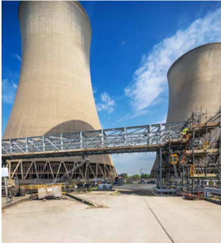
Hundreds of metres of trench covers & frames were required for several trench runs
