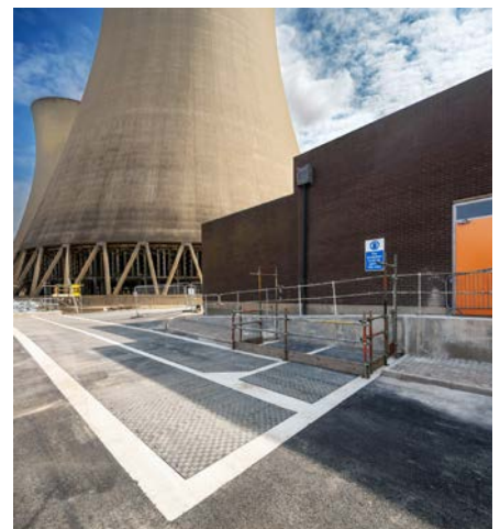
Restraining bolt mechanisms added for added security
