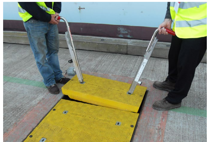
F900 Fibrelite covers installed at the UK's largest port, Felixstowe.
