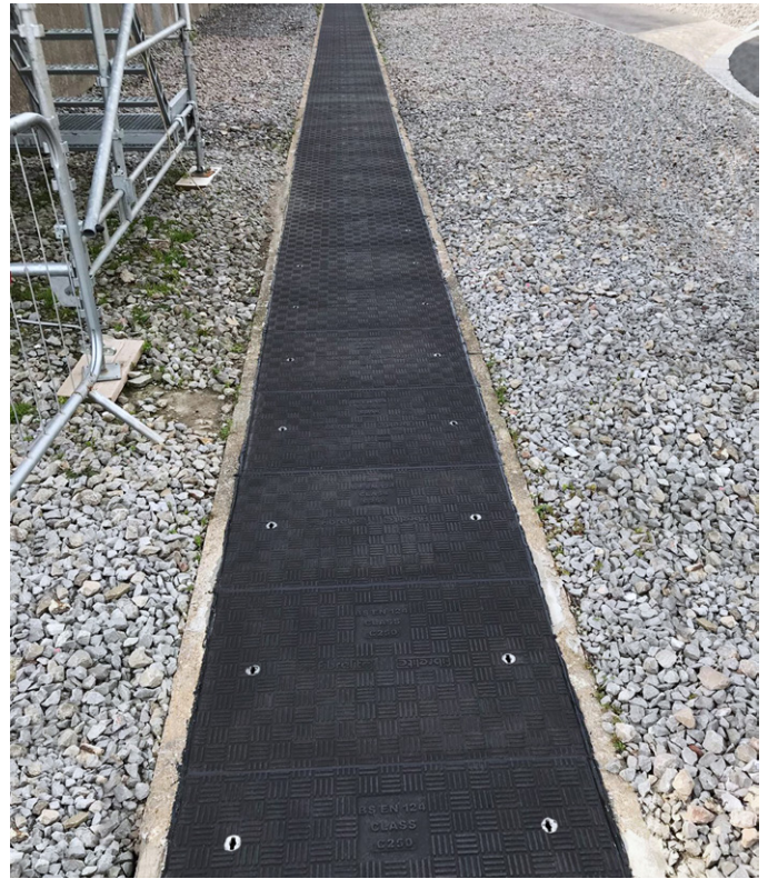
Fibrelite's lightweight covers can be safely manually removed
