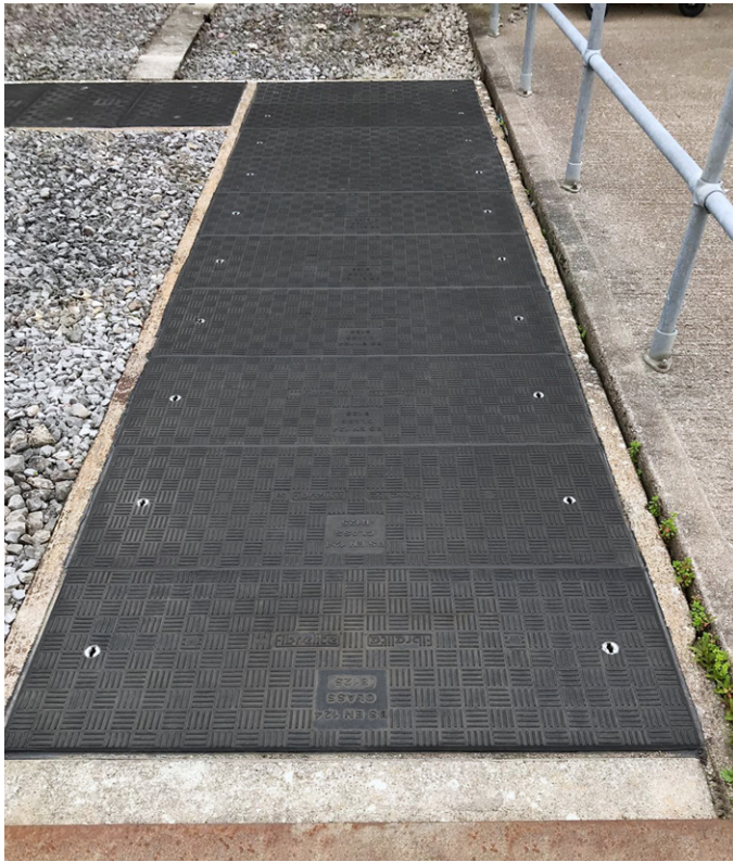
Fibrelite covers are chemically inert and have an anti-slip tread pattern
