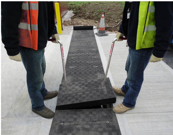
All Fibrelite trench covers can be safely and quickly removed by two people using the FL7 lifting handles (image used for illustration purposes and shows a different installation)
