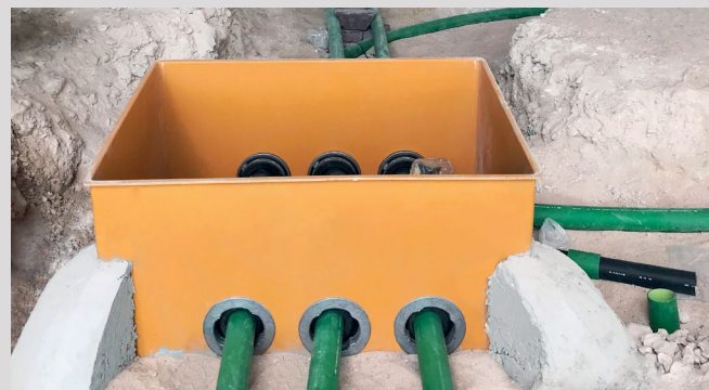
Qatar 20 Site Upgrade Programme
