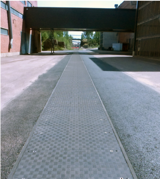
A straight run of Fibrelite FM500-1265-117-D400-2RB panels in between server halls
