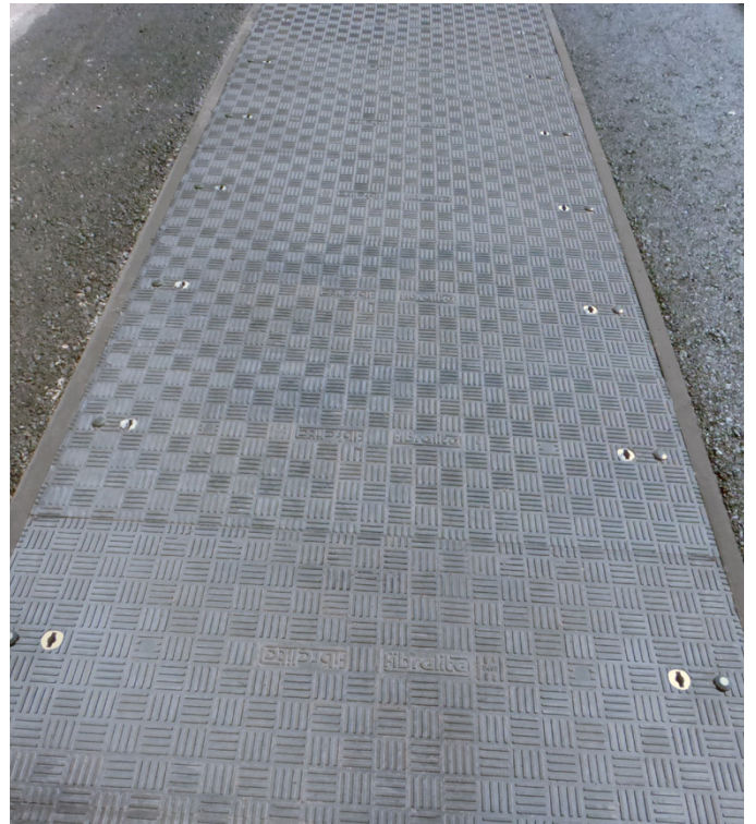
The D400 load rated trench covers capable to withstand heavy duty traffic. Bolts were added for extra security
