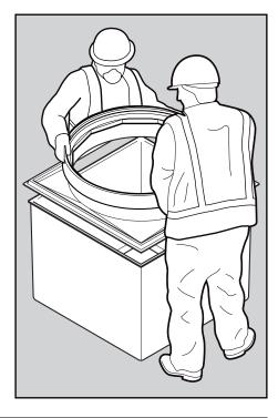
Seal around the inside edge of the corbel joint from inside the chamber. Smooth off the sealant with soapy water.
