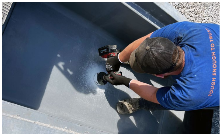
Solid bottom bases: limited openings and drain holes can be field cut
