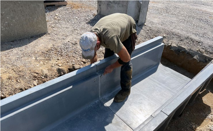
Walls will not flex and do not need bracing during installation and backfilling
