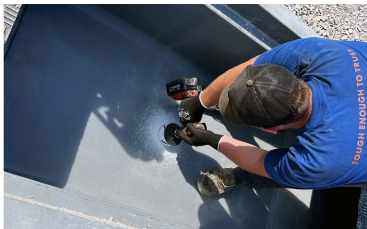
Solid bottom bases: limited openings and drain holes can be field cut
