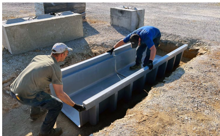
Shiplapped ends for easy alignment
