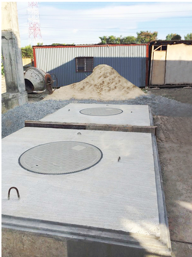
Plinths ready for installation
