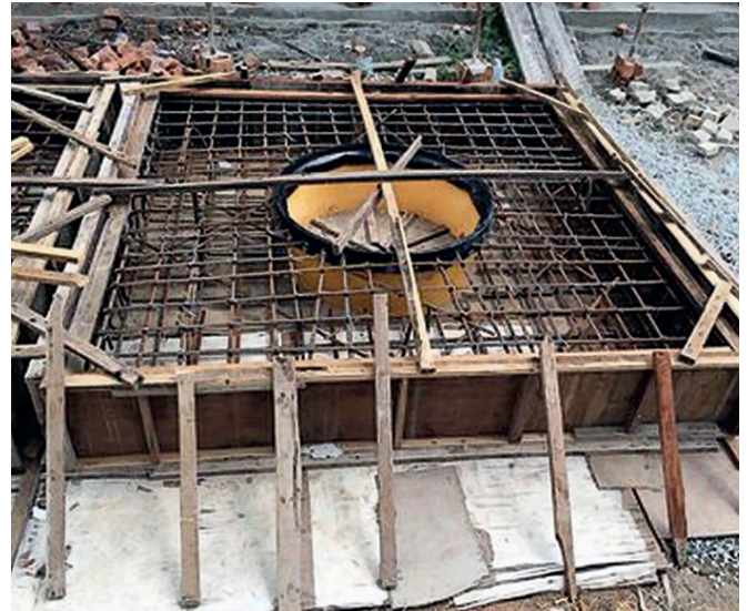
Prefabricating concrete plinth with Fibrelite FL90 frame
