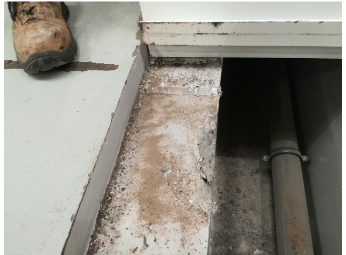
Uneven trench recess depth
