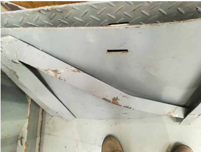
Previously installed covers had also begun to corrode
