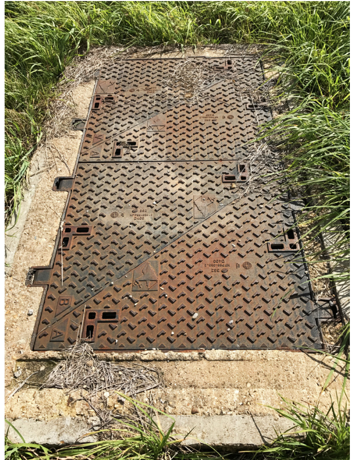
Ease of access to the runway lighting pits off apron was of paramount importance
