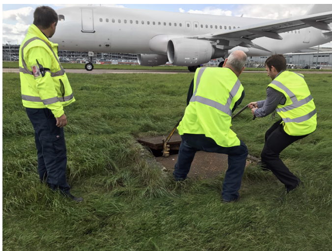
The previously installed cast iron trench access covers were extremely heavy, making them difficult to manoeuvre
