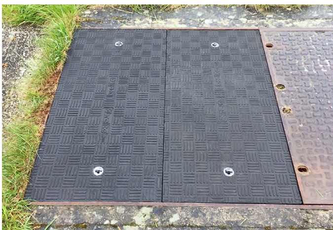
Fibrelite's lightweight F900 load rated trench covers (black covers supplied for fitness check, actual covers purchased were yellow)
