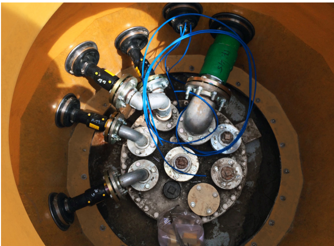
OPW provided a long-lasting containment system
