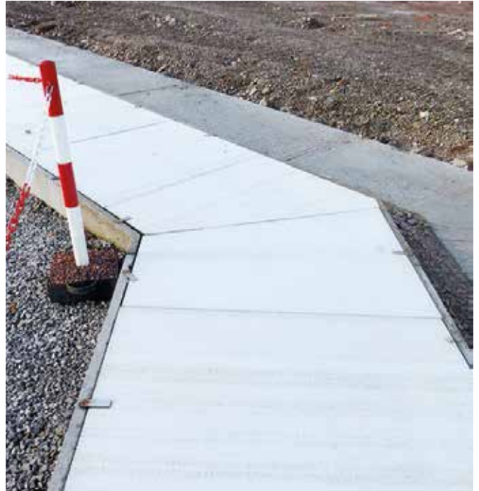
Previously installed low quality concrete covers
