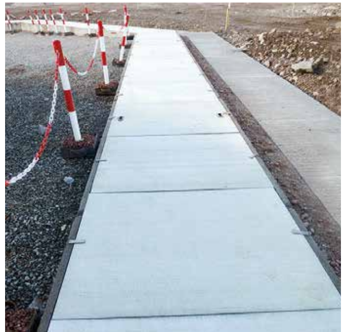
Concrete covers unable to withstand pedestrian traffic
