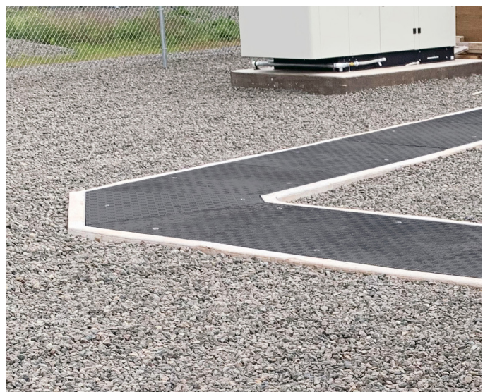
Fibrelite custom engineered an angled trench panel to fit into the existing precast concrete trench
