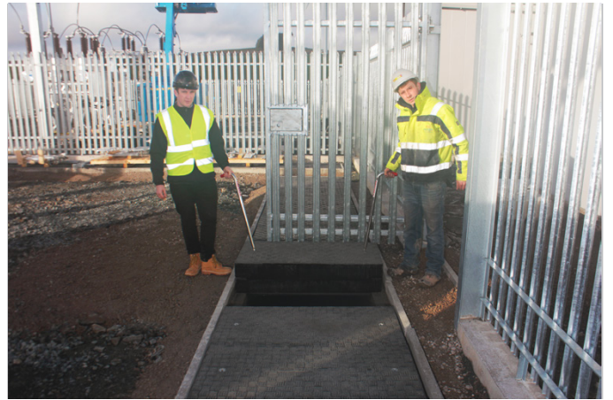
All Fibrelite trench covers can be safely and quickly removed by two people using the FL7 lifting handles (image used for illustration purposes and shows a different installation)
