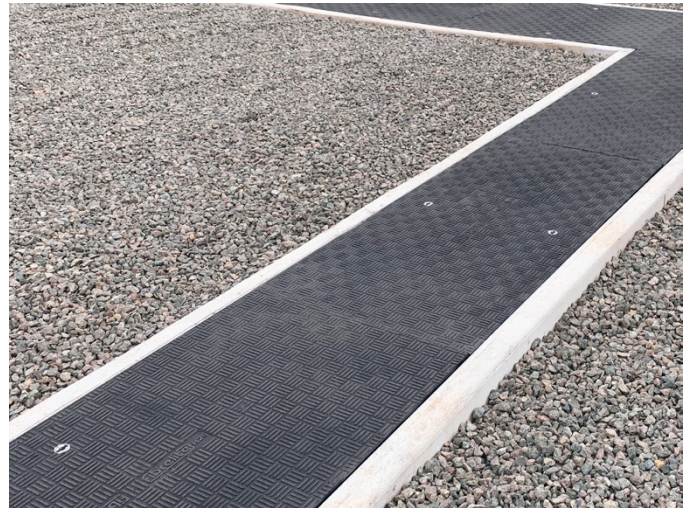
Fibreglass panels weight 2 to 3 times less than their iron and concrete counterparts of the same size
