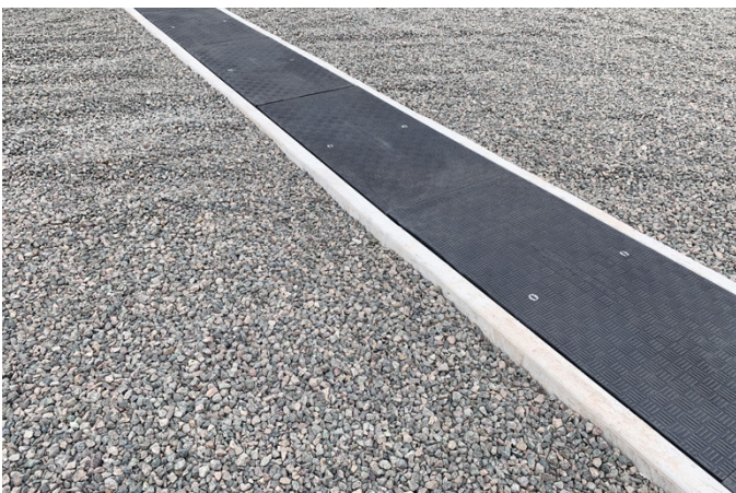
The project needed trench access covers that wouldn't be affected by the corrosive salt and other snow melting chemicals used
