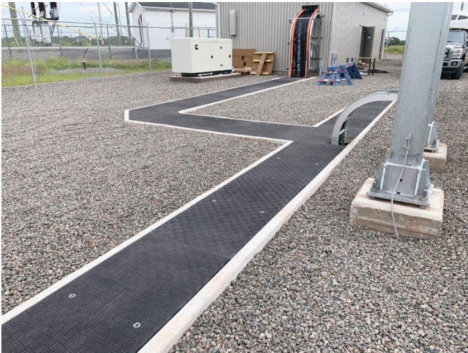
Maritime Electric's new facility on Prince Edward Island required retrofitted trench covers to fit their precast concrete trenches
