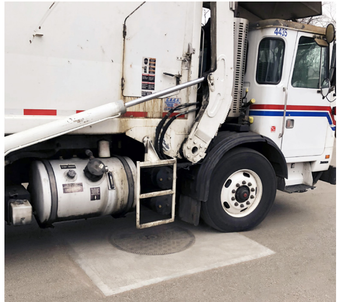
The water company is now installing several hundred additional composite covers with antennas
