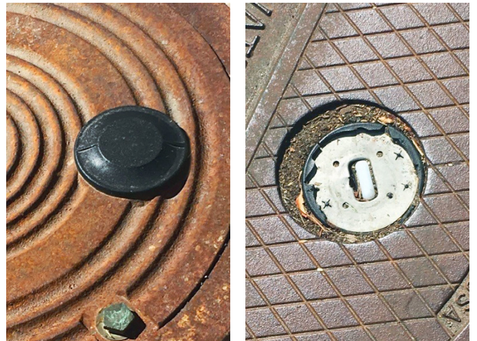
Previously installed metal covers exposed the antenna above the cover in order for the system to work
