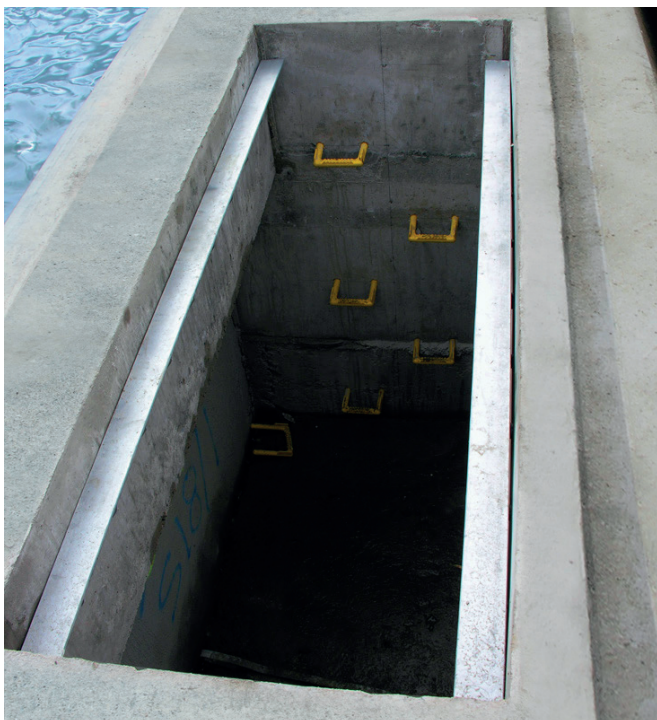
Access pit along edge of quay
