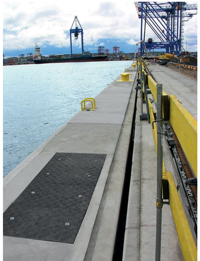
Fibrelite's trench covers covering access pit
