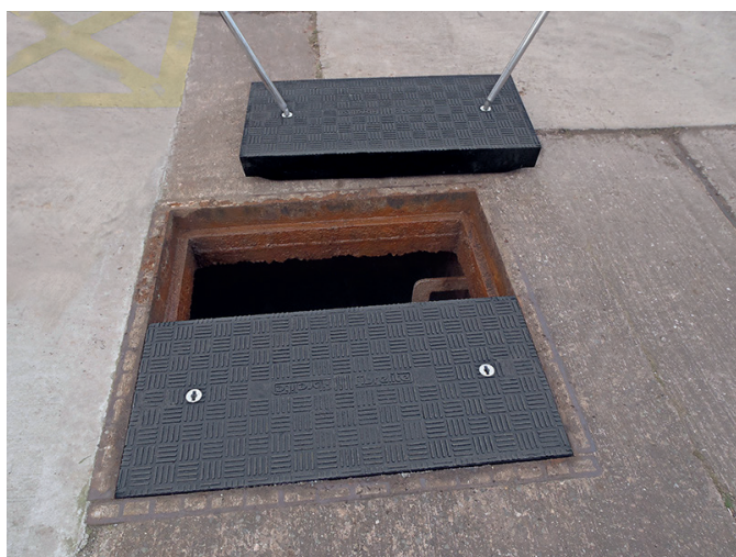
Bespoke Fibrelite covers installed into existing frame
