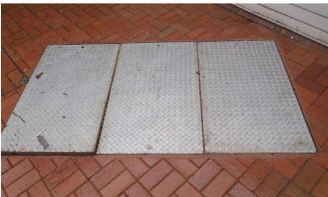
Previously installed odour-emitting galvanised covers
