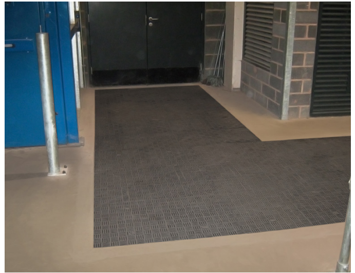
Fibrelite's trench panels can be used to cover large areas and corners
