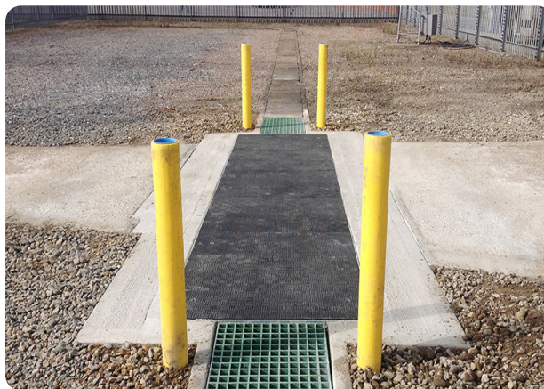
Lightweight composite trench covers
