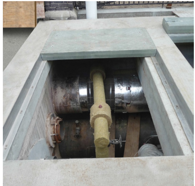
Six Fibrelite FM45 4' 6" (1.6m) wide anti-slip FRP composite trench panels being installed in the sidewalk
