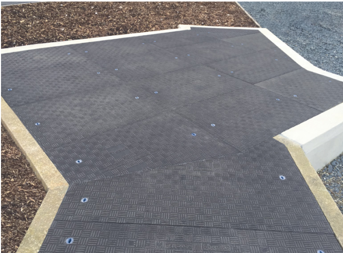
"Cassette" of bespoke covers over culvert
