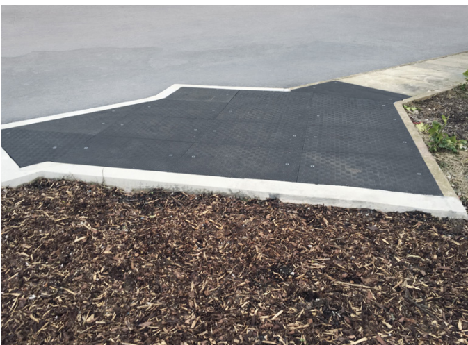
Bespoke "cassette" of Fibrelite covers and supporting steelwork installed to tight construction deadline
