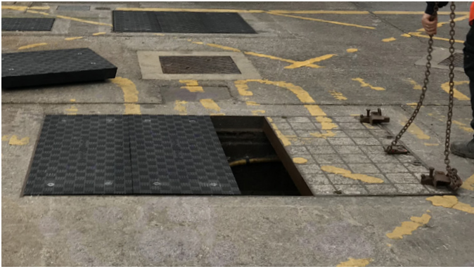
New custom Fibrelite covers engineered to fit directly into existing frames
