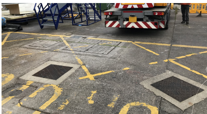
Heavy cast iron recess covers with concrete infill
