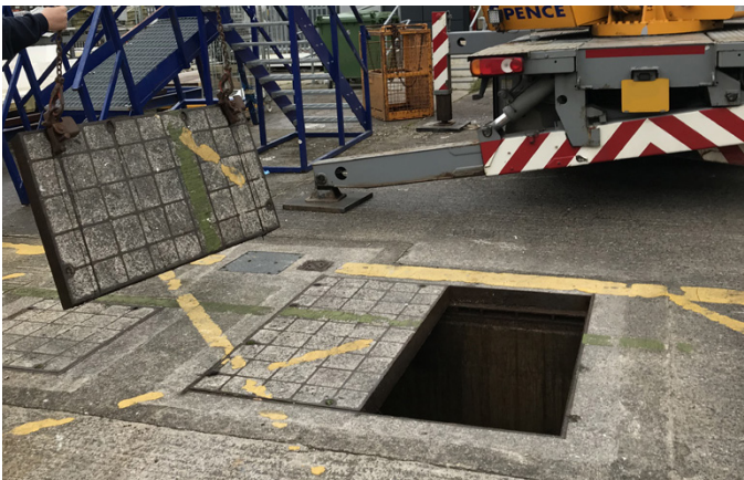
Site managers decided the health and safety risks posed by these heavy cast iron recess covers was no longer tenable
