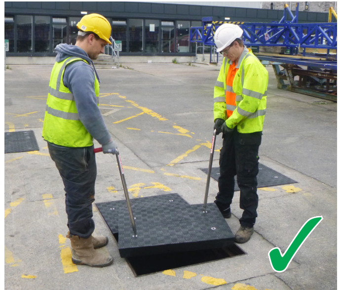
Fibrelite's lightweight composite covers can be safely removed and replaced by two people
