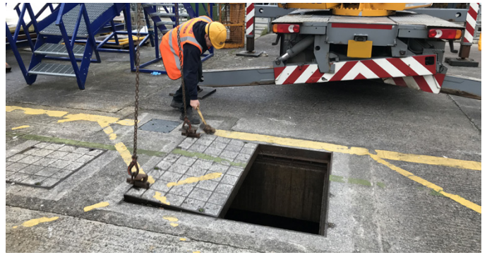
Existing key housings had corroded/deformed adding to difficulty incurred during removal
