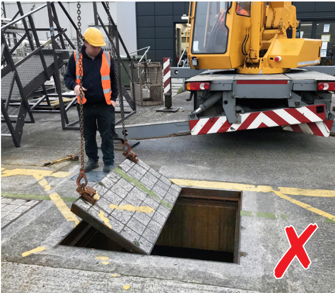
Previous installed access covers required a crane to remove and replace
