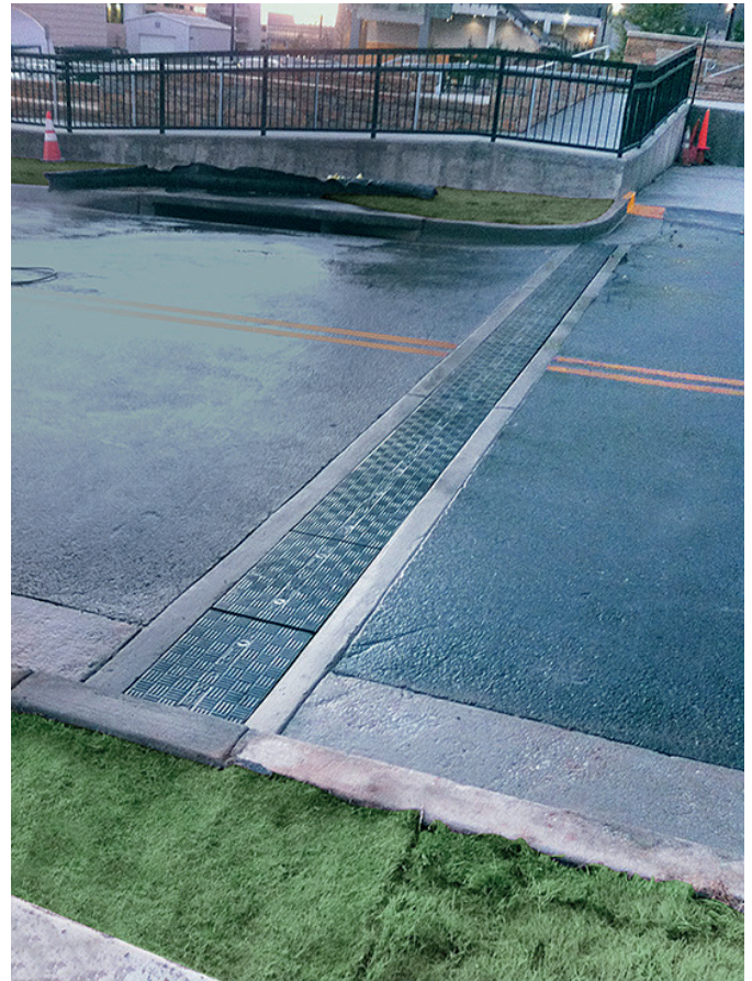
Fibrelite covers offer a clean lightweight alternative to heavy and iron concrete covers
