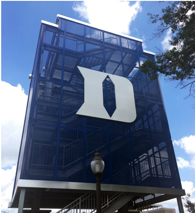
Duke University install Fibrelite trench covers
