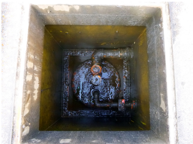
Previously installed chambers allowed water ingress
