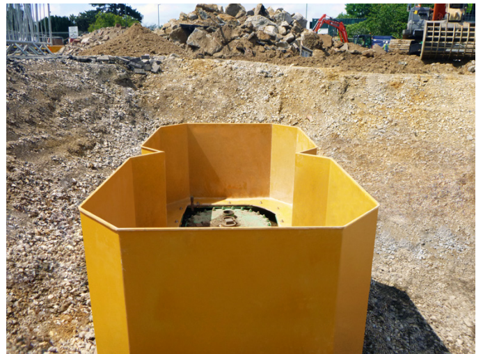
The new double chamber fit to the previously installed split container tanks
