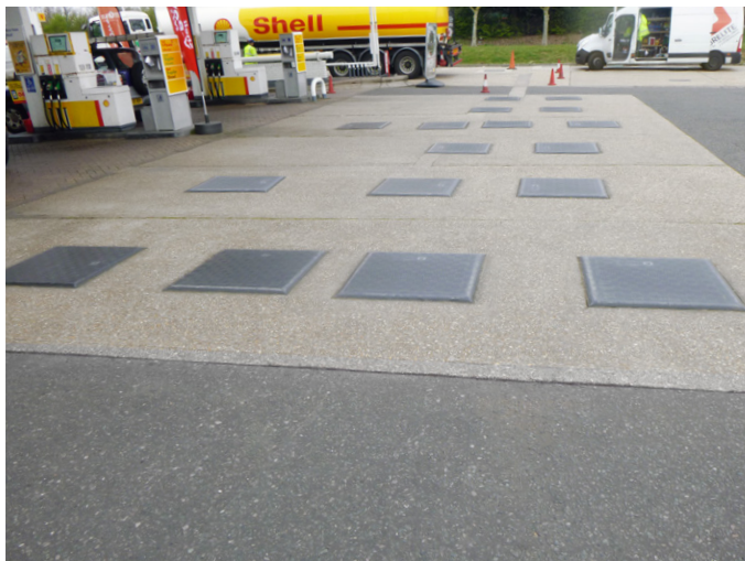
Unusual site configuration with double tank manways
