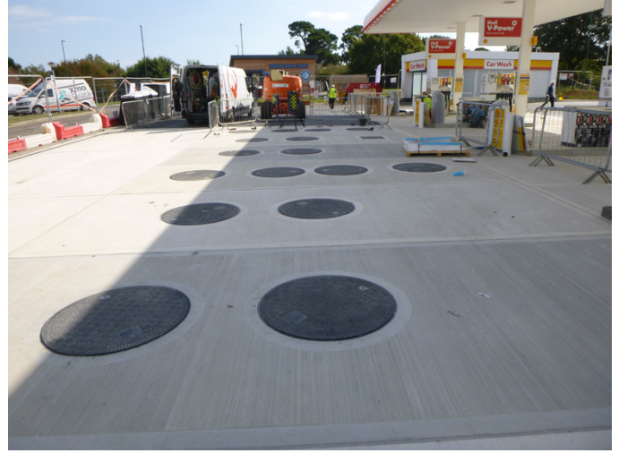
Fibrelite's composite manhole covers appear bunched together on the surface to cover the joint chambers
