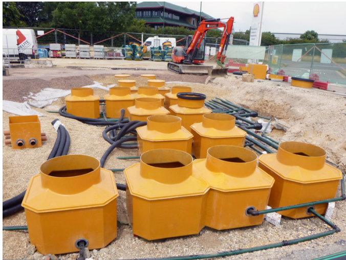
Bespoke Fibrelite chambers installed at Shell Eastfield
