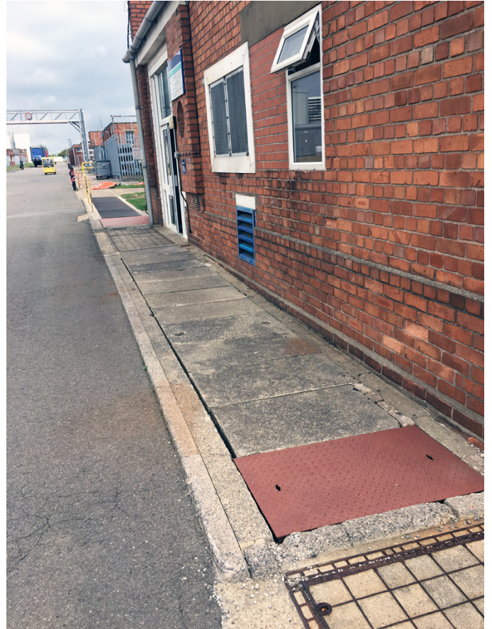
Previously installed covers had cracked and corroded
