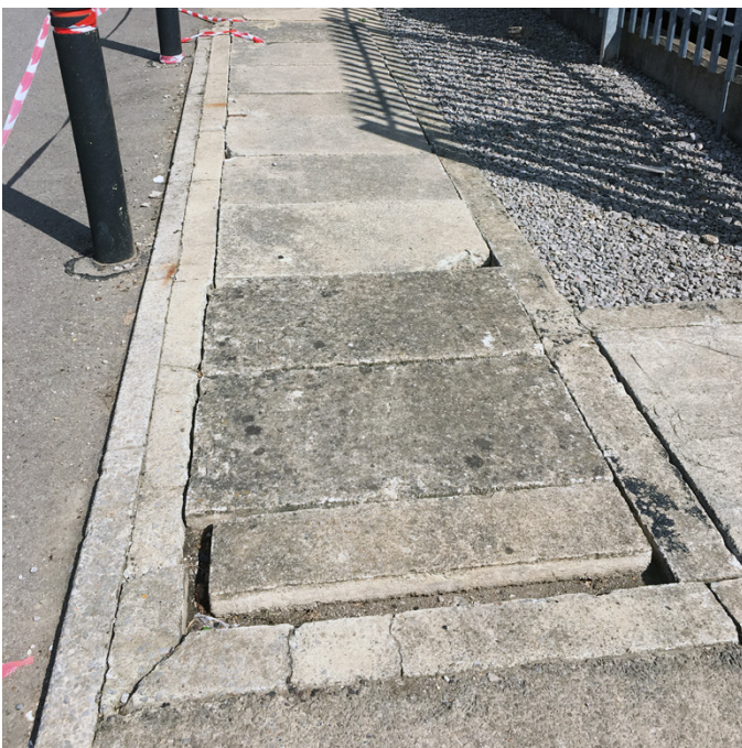
Previously installed failing concrete trench access covers
