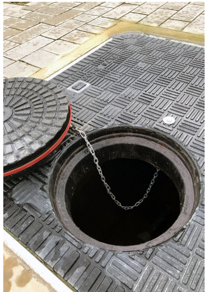
The Fibrelite cover that was installed can be easily removed by one person
