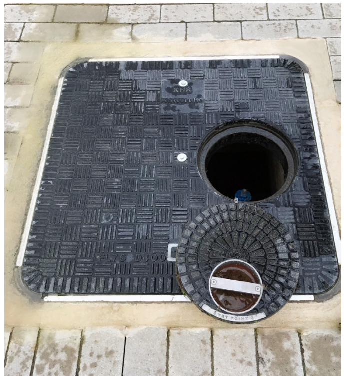
Fibrelite covers are corrosion-resistant, unlike metal covers
