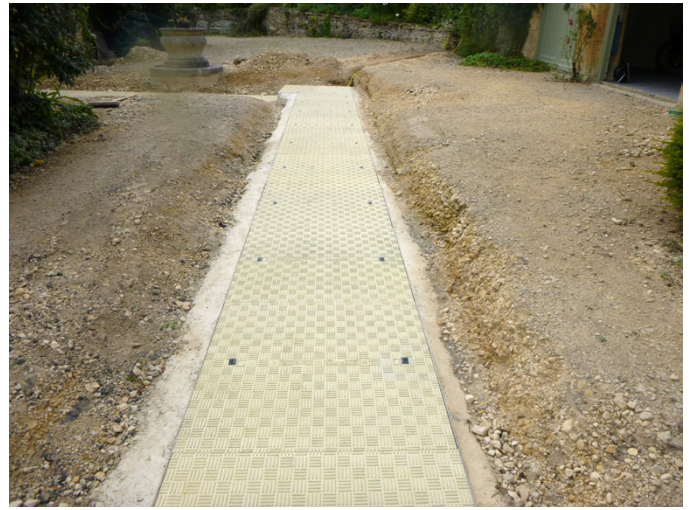
Fibrelite covers can be safely removed manually by two people
