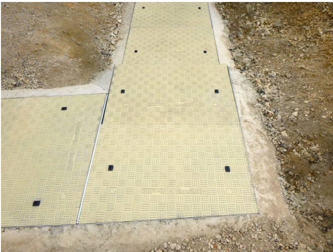
Fibrelite custom manufactured trench covers in a colour that blended in with their surroundings
