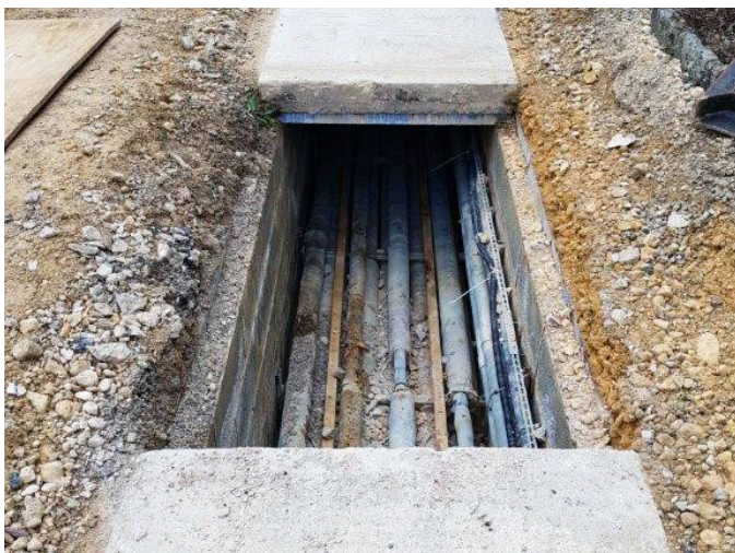
Fractured covers had allowed dust and debris to enter the trench
