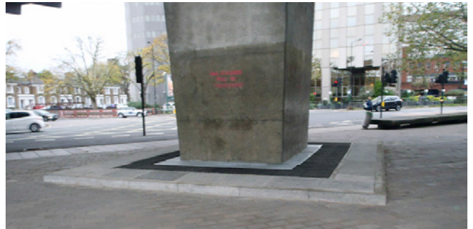
Roller bearings at the bases of supporting piers were replaced due to wear and increased load on the bridge
