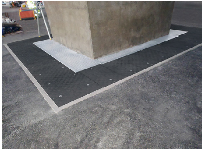
Replacement bearings located in the underground pits, covered by continuous set of access covers, allowing for the minor movement of the pier
