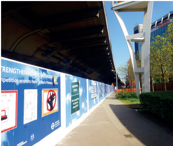
London Hammersmith flyover during refurbishment
