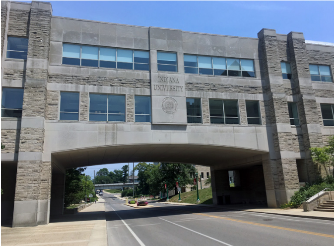
Indiana University required steam rated manhole covers
