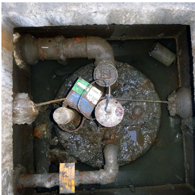
At this site, the old tank upstands were too small for the traditional bolt down chambers tank sumps / chambers
