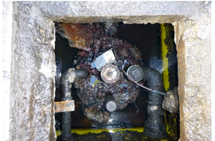
Shell required a retrofit watertight solution
