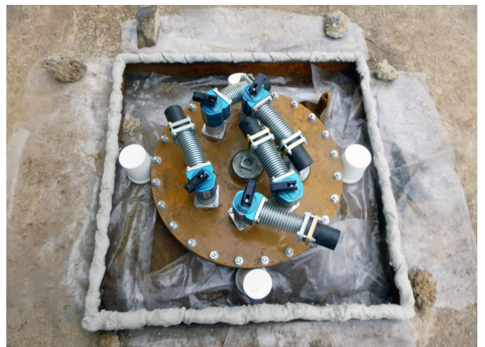
Preparation of surface for putty
