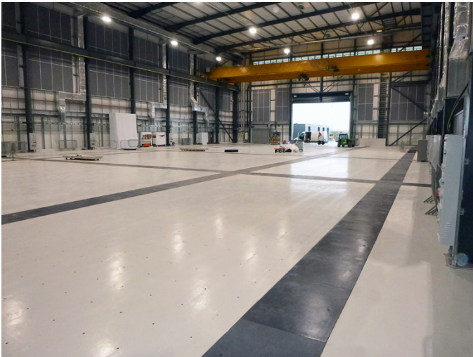
Fibrelite provided a bespoke composite trench covering arrangement for this manufacturing and research facility
