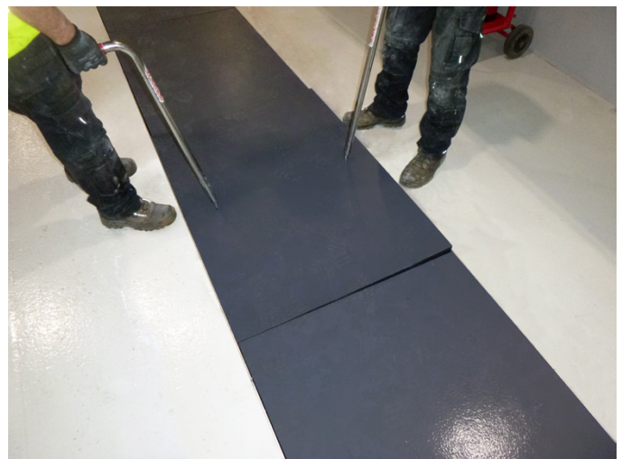
All Fibrelite trench covers can be safely and quickly removed by two people using the FL7 lifting handles
