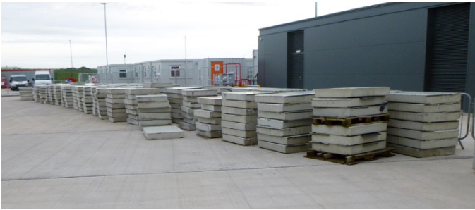
Previously existing concrete covers stacked, awaiting disposal
