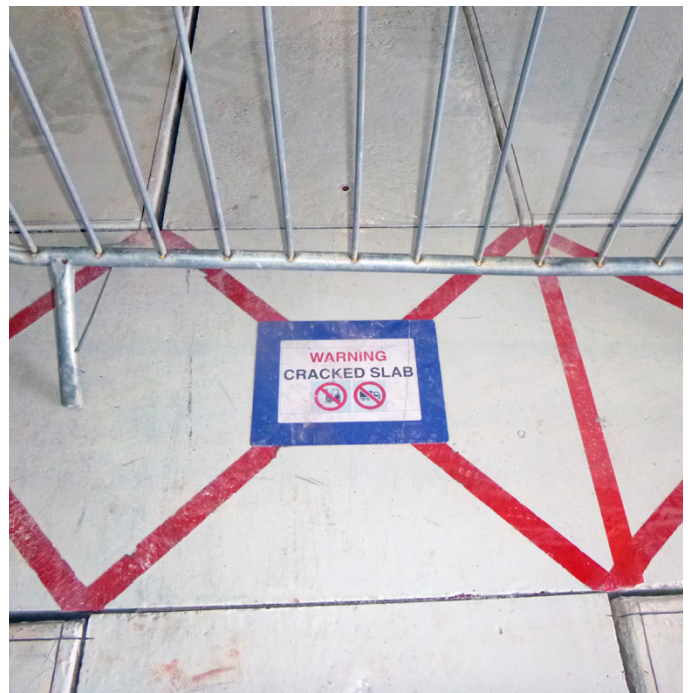
Previously existing D400 concrete covers were cracked in some areas
