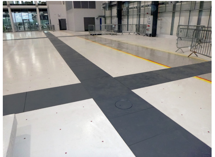
Fibrelite trench covers are designed to be safely removed manually
