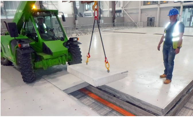
Removing the previously existing covers was a costly and time-consuming operation
