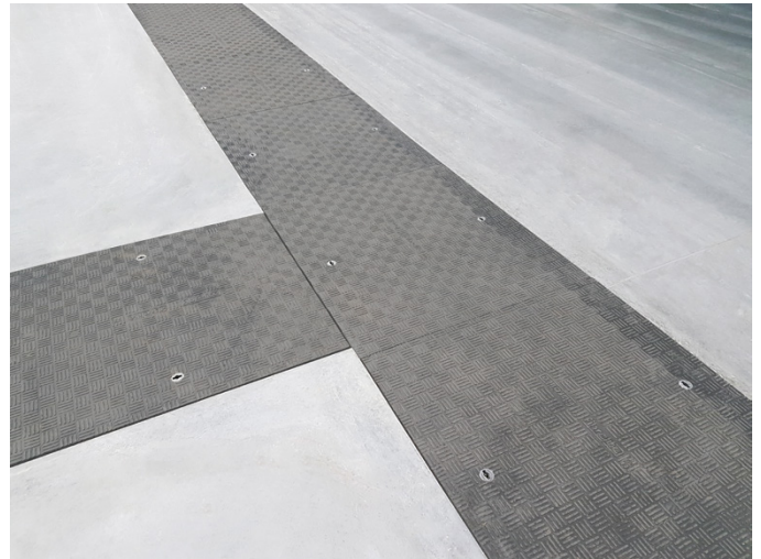
Fibrelite and Corrimex installed a T junction as a part of the project
