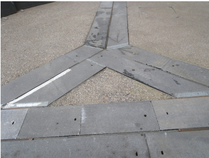
Existing covers had no tread pattern, potentially causing their surface to become slippery when wet
