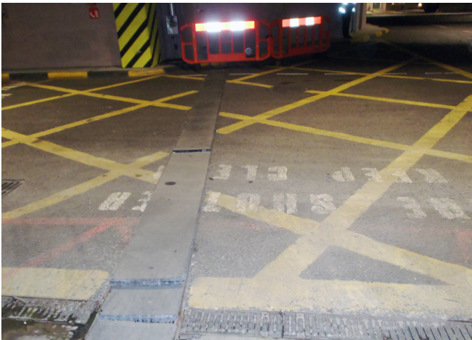
Previously installed covers were poorly fitting in their frames due to the covers being distorted.
