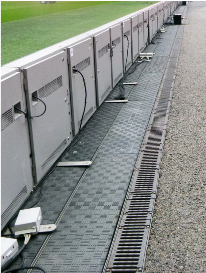
Lightweight Fibrelite covers allow easy, safe removal by 2 people
