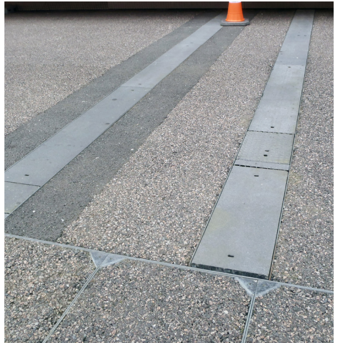
Previously installed covers were unable to withstand heavy loads causing them to crack and deform
