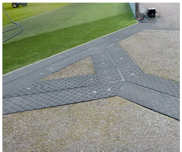
Fibrelite covers are chemically inert so will not corrode over time
