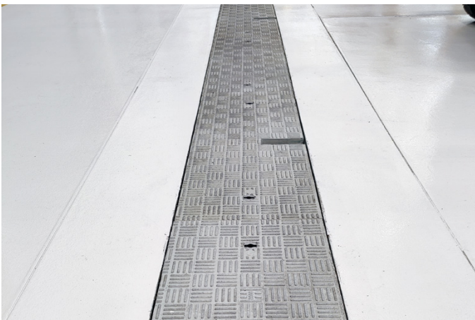
A E600 'Super Heavy Duty' load rating was essential due to the frequent high wheel loads
