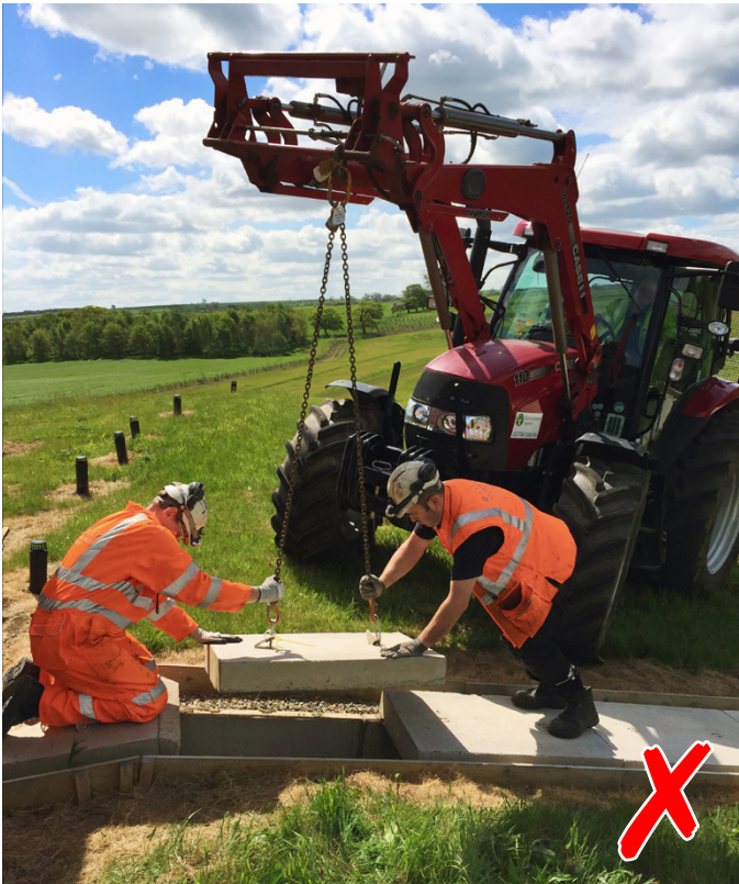
Heavy duty lifting apparatus had to be used to remove and replace the existing concrete covers
