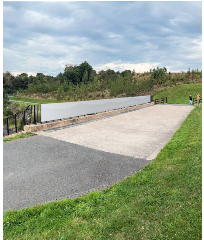
It was essential for the new trench covering arrangement to be retrofitted, lightweight and easy to use
