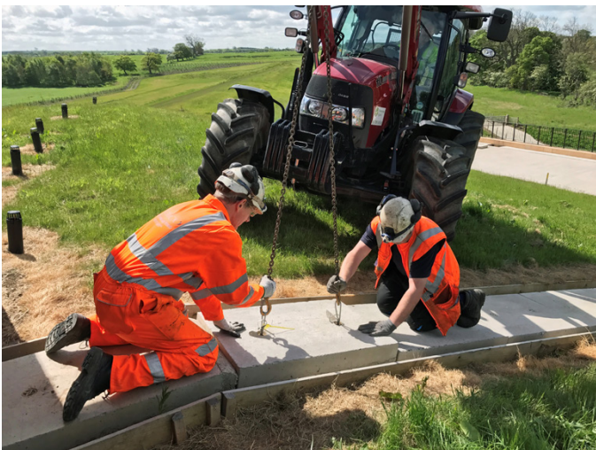
Specialist training was required for operatives to remove and replace the previously existing concrete covers
