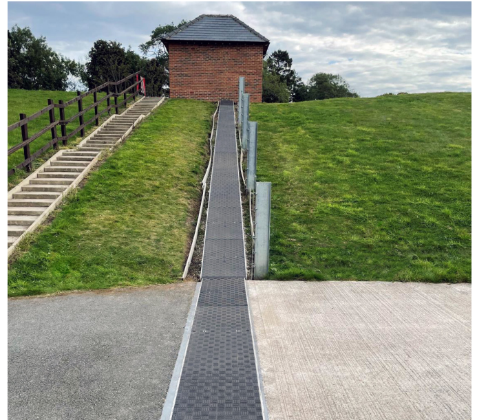
Bespoke C250 and A15 load rated covers supplied in line with client requirements
