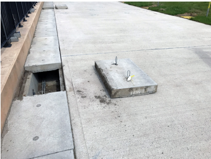
Heavy duty lifting apparatus was required to remove and replace existing covers
