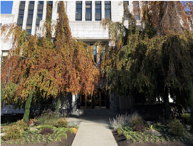
Fibrelite provided lightweight retrofit trench access covers to Vancouver City Hall
