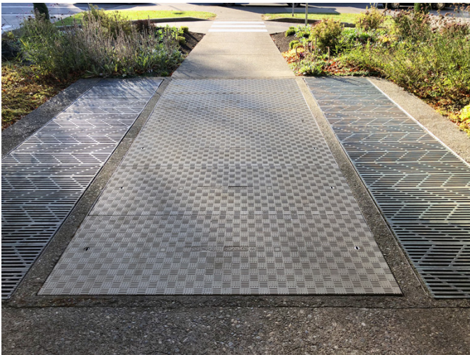
Fibrelite covers allow quick safe manual removal
