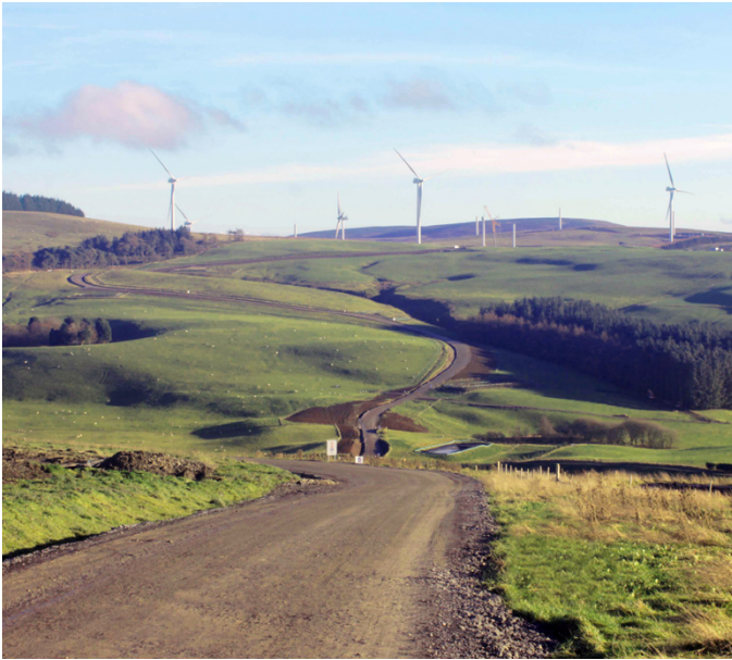
Garreg Lwyd wind farm under construction
