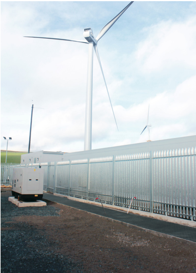
Fibrelite D400 trench covers on wind farm substation
