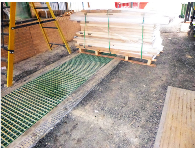
Previously installed GRP grating was originally supplied together with the precast concrete troughs
