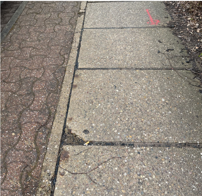
The previously installed concrete covers had begun to deteriorate
