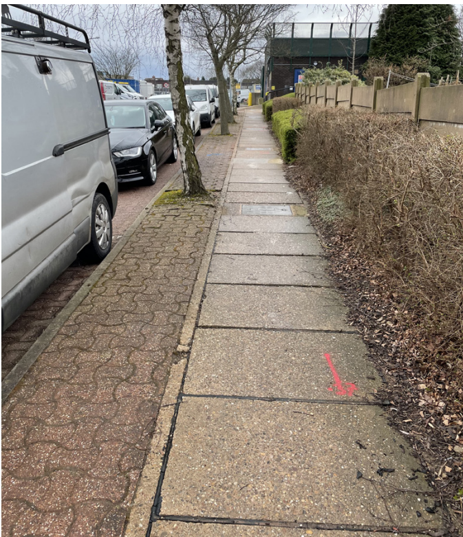
The previously installed heavy concrete access covers had cracked
