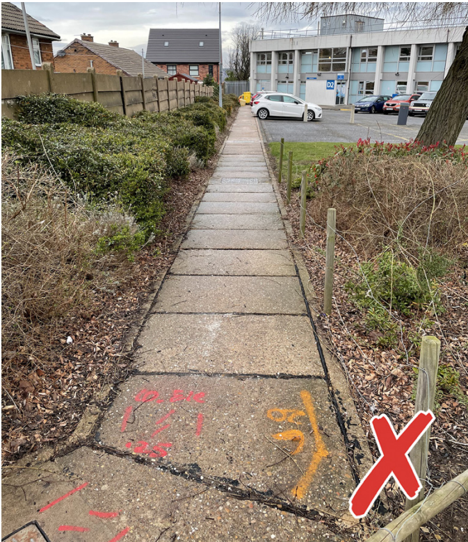
Previously installed heavy concrete trench access covers
