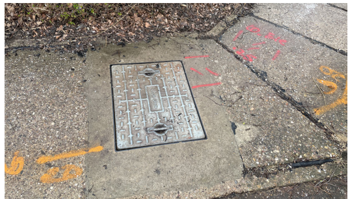
A bespoke replacement was required for the previously installed access covers
